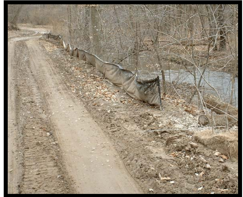
Silt-fence application.
