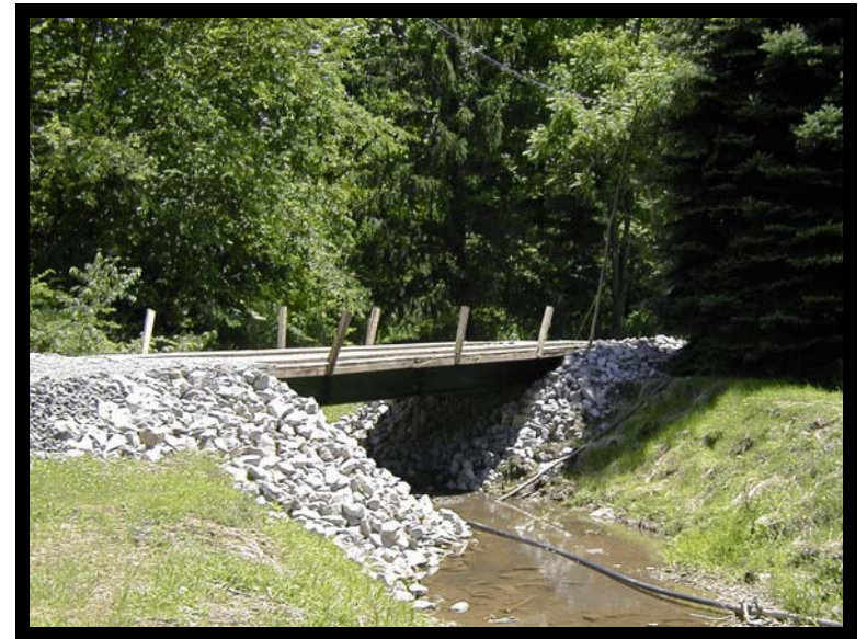
Portable temporary bridge.
