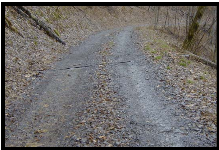
Open-top pipe culvert.
