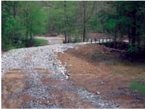
Haul road bridge
