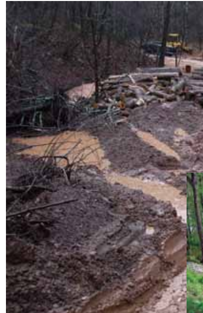
Poor landing location
