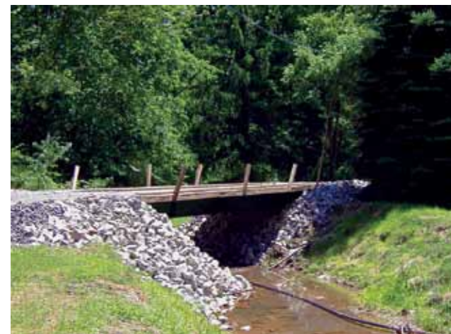
Temporary bridge installation in SMZ
