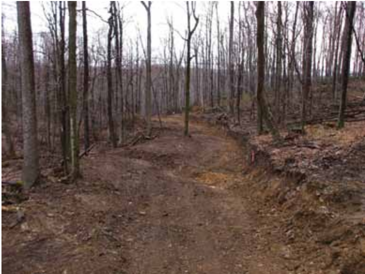
A good water bar. Note outflow end is open and proper construction angle across road.
