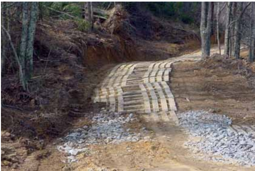
Haul road with use of timber mats for stabilization.
