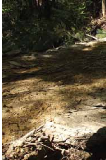
Simple but effective skid road bridge
