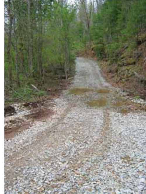
Haul Road fording creek. Note significant limestone surfacing.
