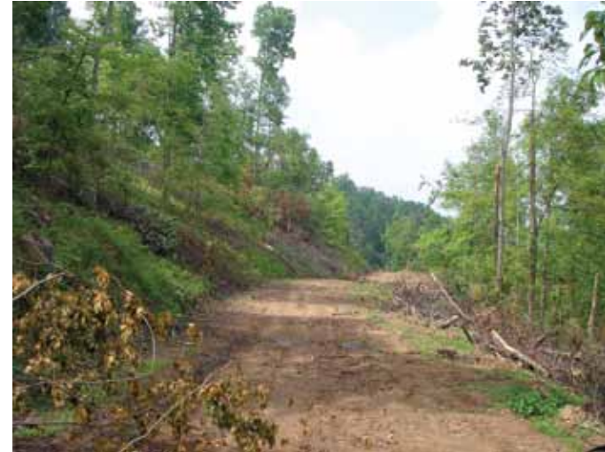
Well-constructed skid road
